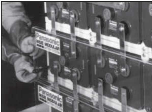
Figure 5.4 Attach safety shield with fastening nuts
