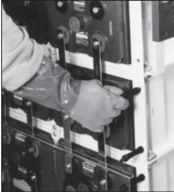
Figure 5.3 Attach four shield standoffs by hand
