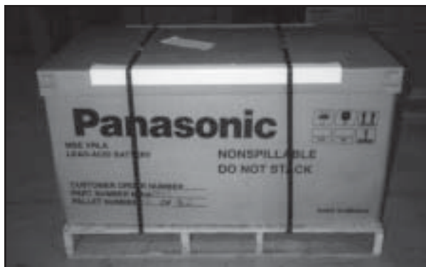
Figure 3.1 Inspect boxes during delivery
